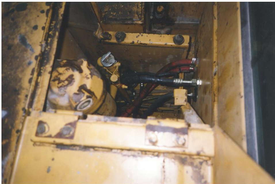
Drier in place with hoses.
